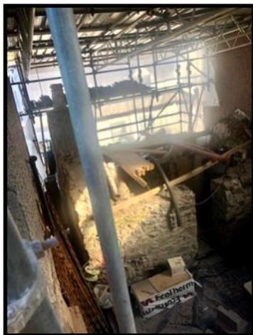
The old Ferryman's Cottage on Beach Road is undergoing change! In the photo you can still see the chimney on the left and a blocked up window at the back has been made into a doorway. The roof has been removed and will be replaced using as many of the old small slates as possible. Hard to say what was holding the roof up really, all the roof rafters were rotten. The front of the property and the one room
